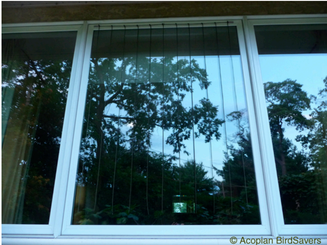
This photo and the one on the next page are from the Acopian BirdSavers website and show DIY installations. Here you get a bird's-eye view.
